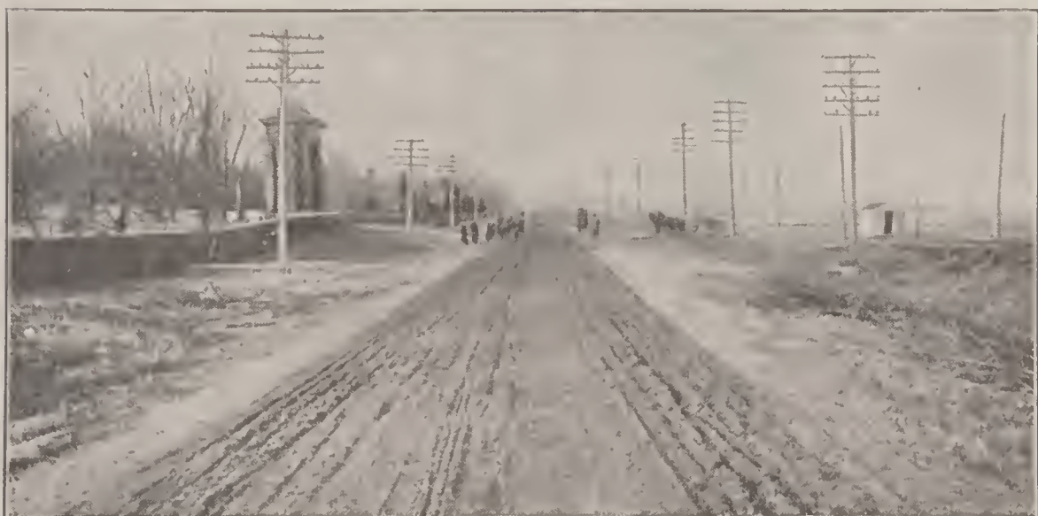
Road before Dragging
